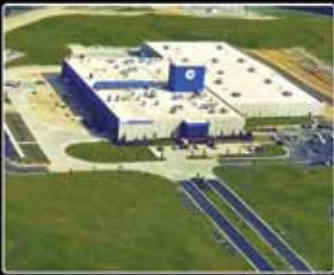
PAGELAND, SC Bronze Foundry and Manufacturing Plant
