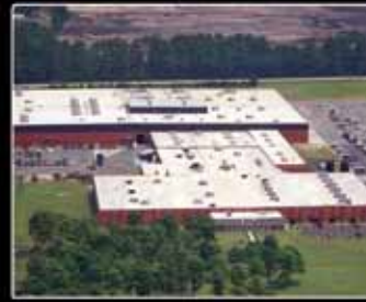
CONWAY, SC Steel Foundry and Manufacturing Plant
